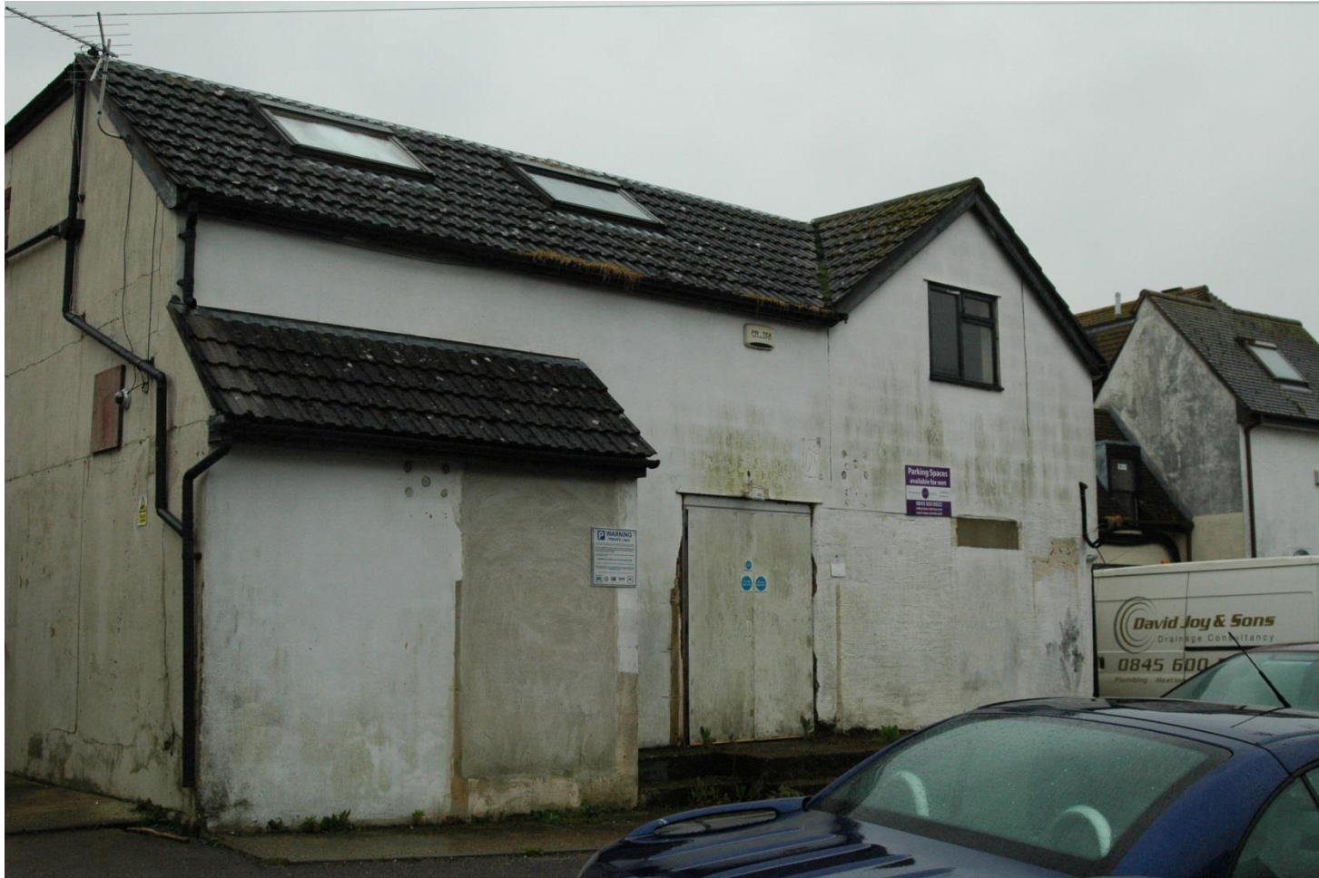
Rear elevation - before
