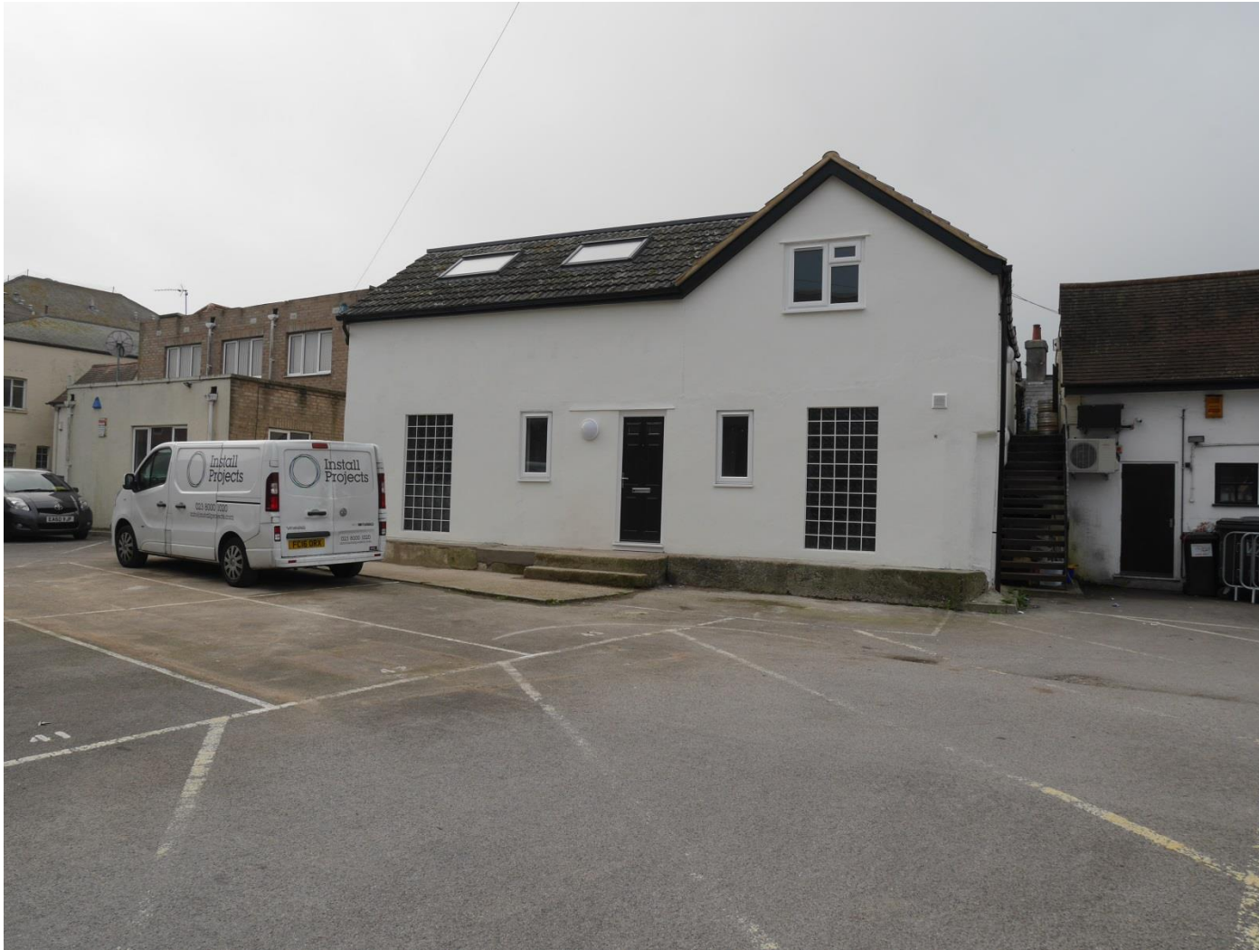
Rear elevation - after
