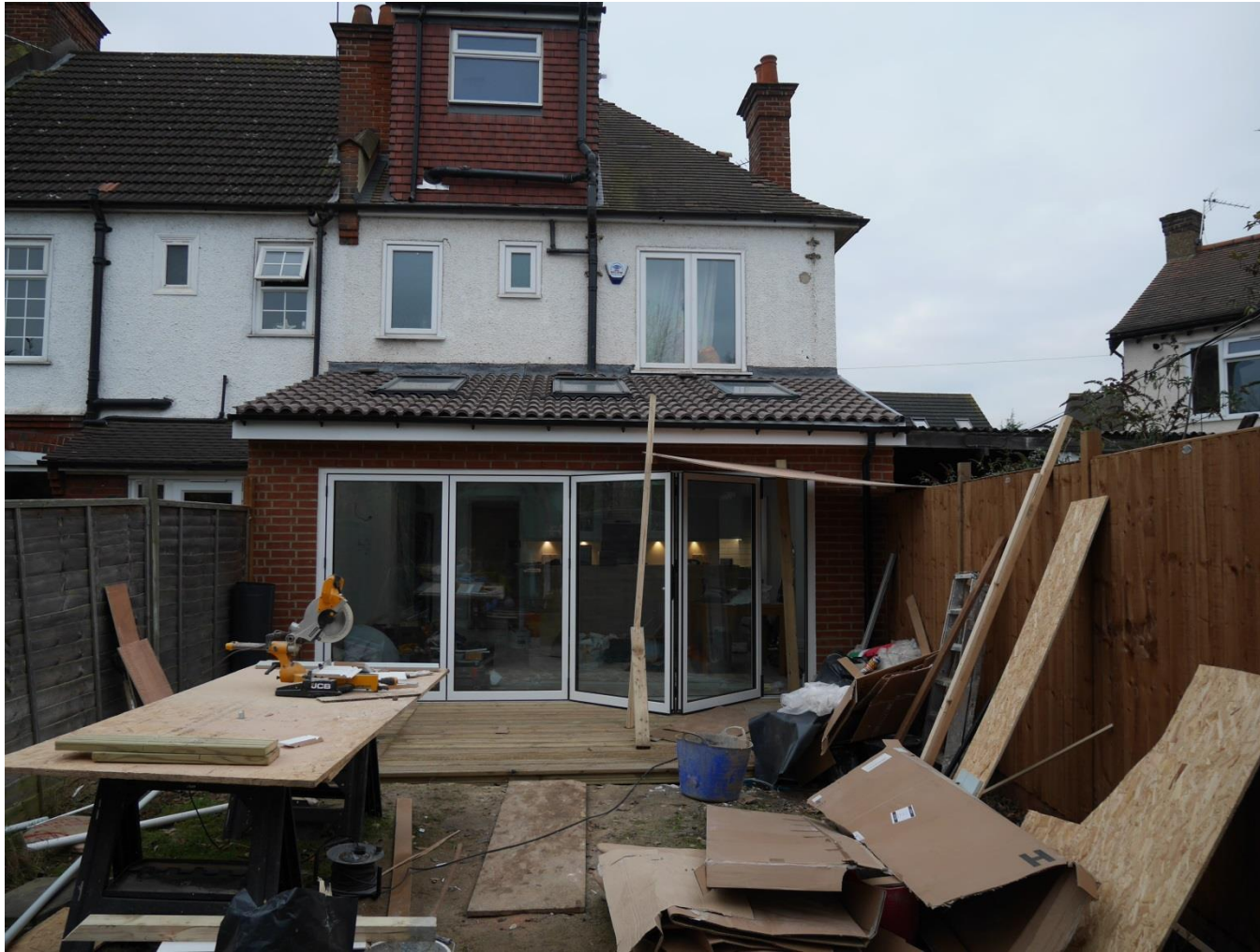
Rear elevation after
