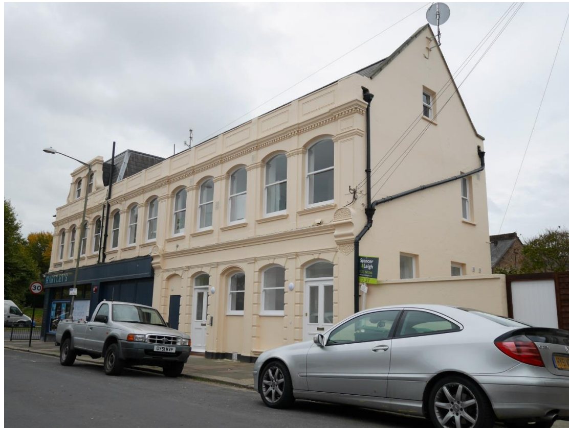
Flank elevation - after
