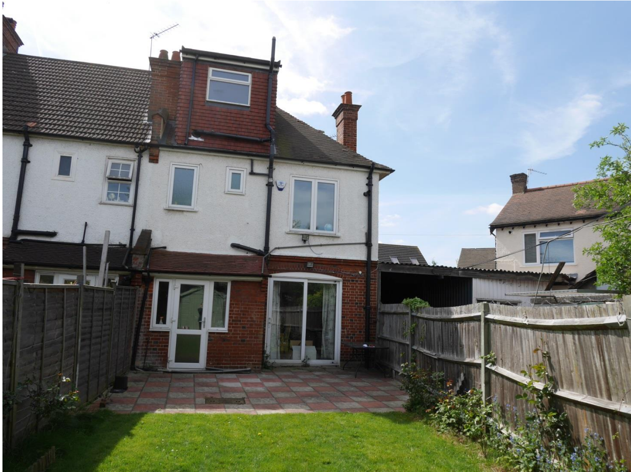
Rear elevation before
