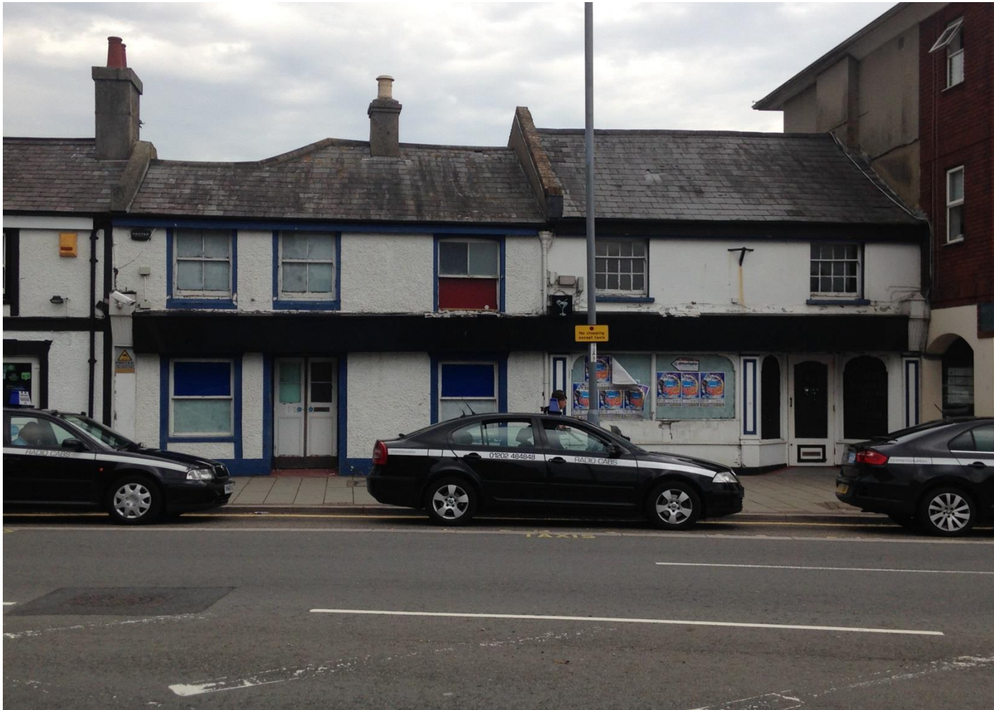
Front elevation - before
